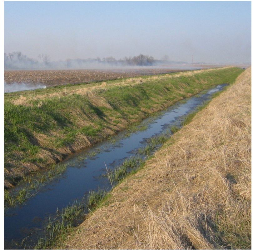
Surface drains (ditches)
