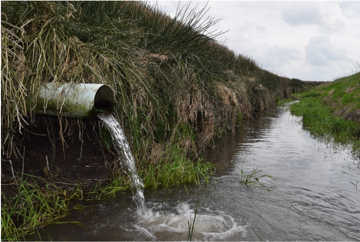
Subsurface tile drains
